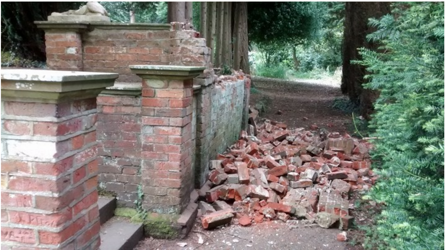
Terrace wall pushed over August 2016
