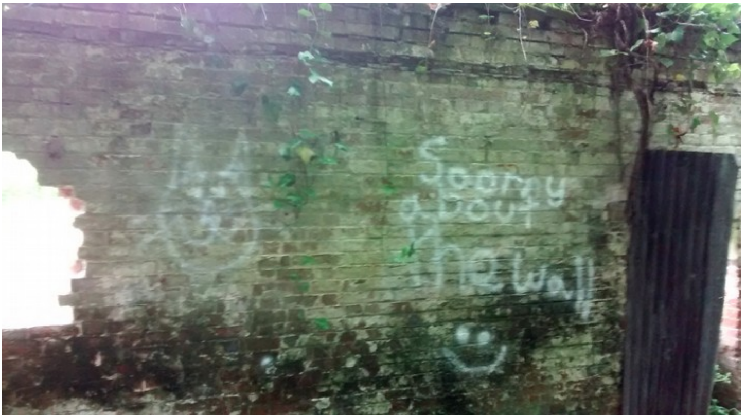
Wall damage – bricks removed and graffiti over a period of time
