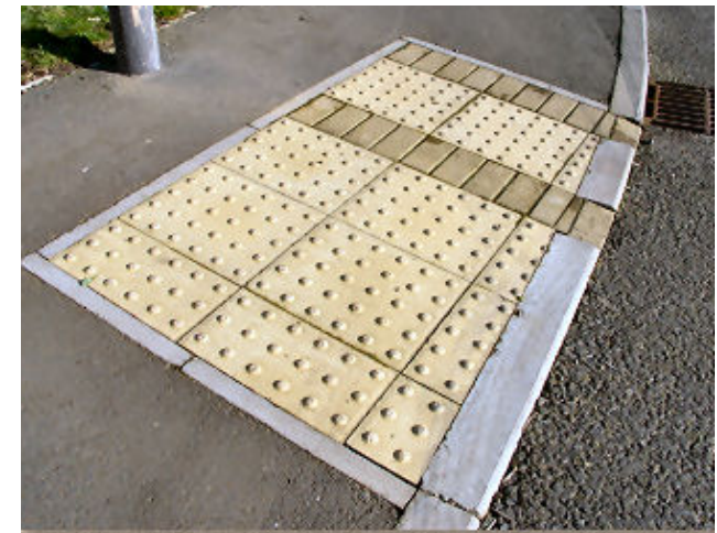
Example of Tactile Paving
