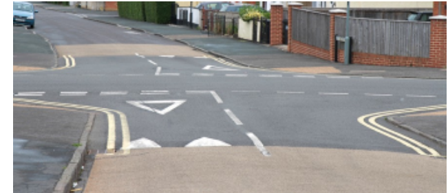
Example of Raised Tables
