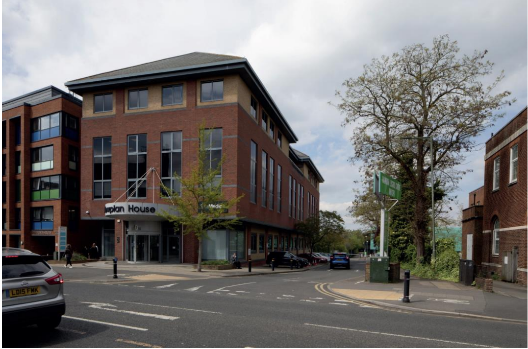
Figure 36: East Street/New Plan House Existing
